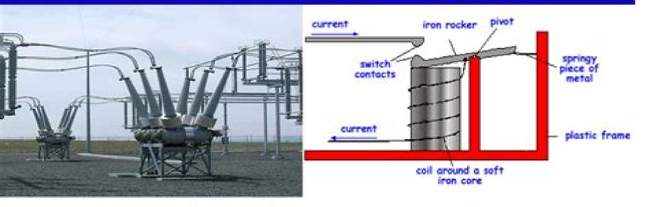
A circuit breaker is a switching device that interrupts the abnormal or fault current. It is a mechanical device that disturbs the flow of high magnitude (fault) current and in additions performs the function of a switch. The circuit breaker is mainly designed for closing or opening of an electrical circuit, thus protects the electrical system from damage.
